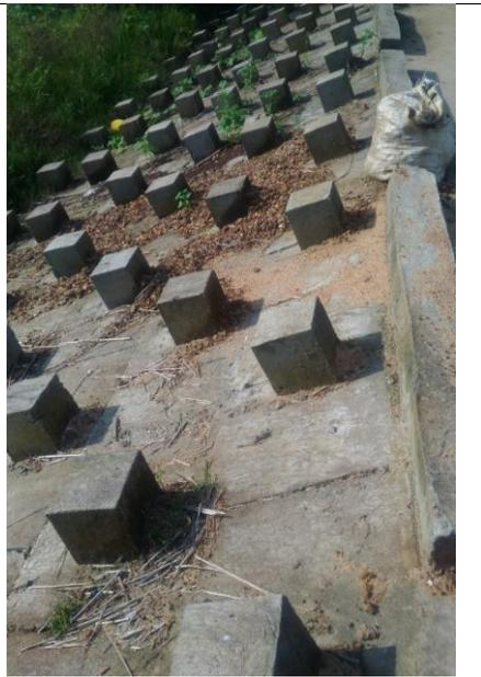
Figure 56: Wave breaker (country side) provided on spill zone located on Damodar Right Embankment at Shibani para
